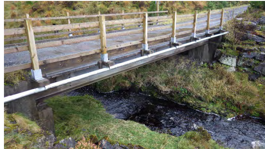
Existing bridge structure
