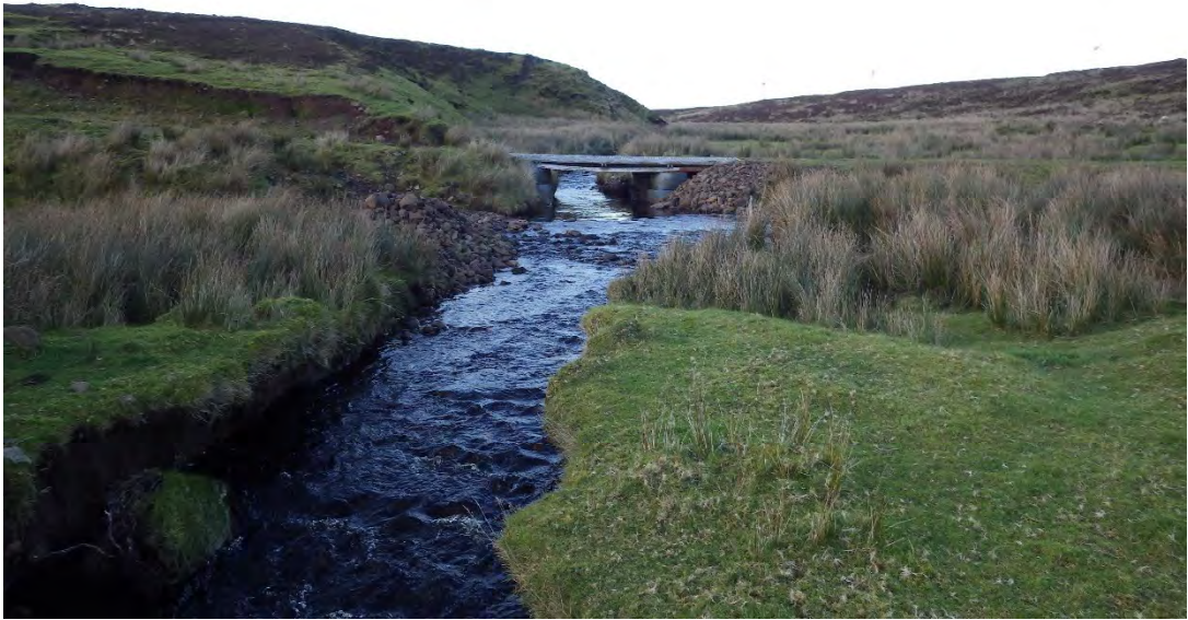
Photograph 9.4.1 View of existing crossing showing cobbles dredged from the channel to either side of the bridge. View N from NGR NG 3071 4695.
