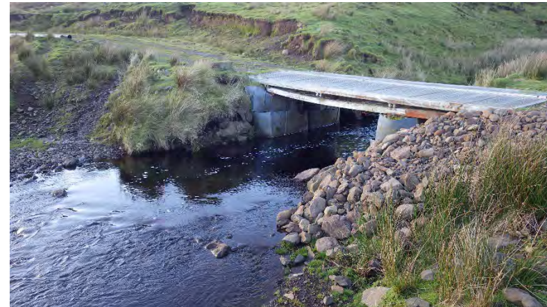
Existing bridge structure
