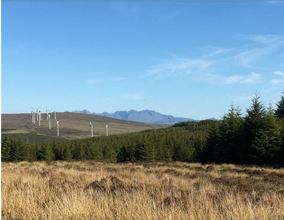
Above: Photograph of the existing Ben Aketil Wind Farm
